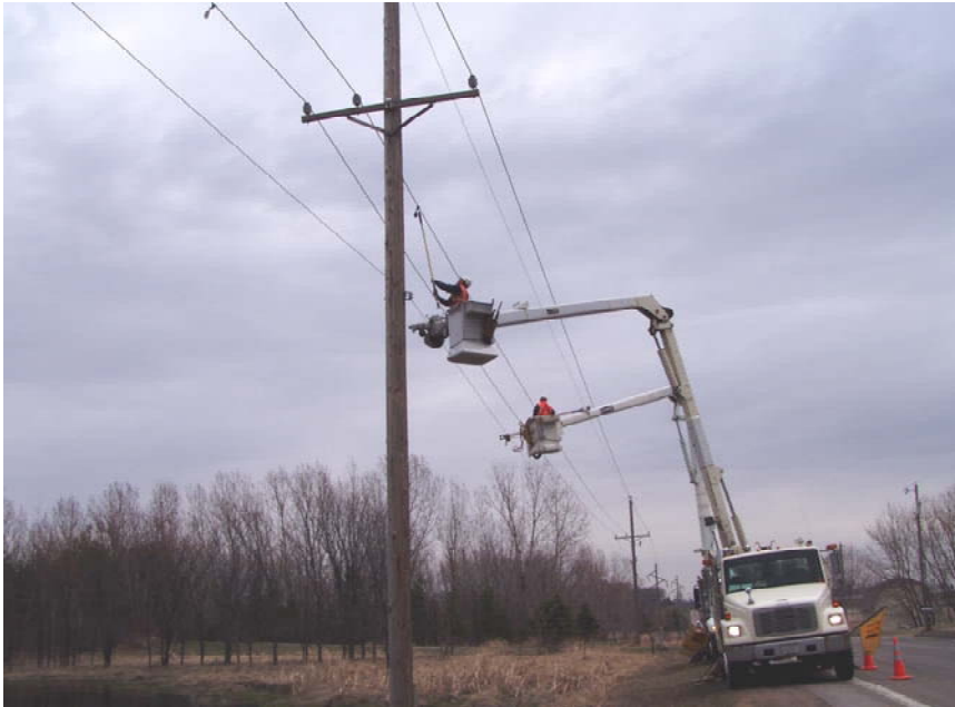
Figure 3. Local energy cooperatives and Xcel Energy install bird flappers on power lines.
